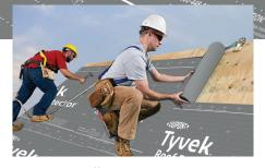
**Easy to Install** Lays down flat and easy to reposition.
